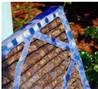
Samples of mold in an AHU (above) and on a Pleated Air Filter (right)
